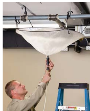
STEP 4: Click drainage hose into place and position toward a drain or collection container.
