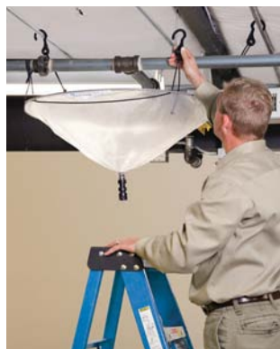
STEP 3: Hang diverter by the hooks and slide it along the straps to level.
